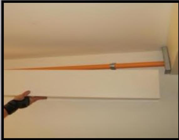
6. SNAP MATERIALS ONTO SHIELD CLIPS
