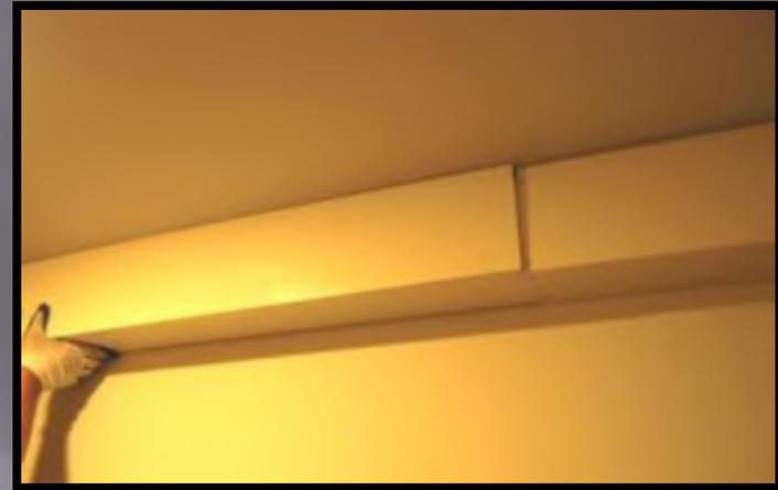
7. DRILL & RIVET THROUGH INTERIOR COUPLING BY MATERIAL SEAM
