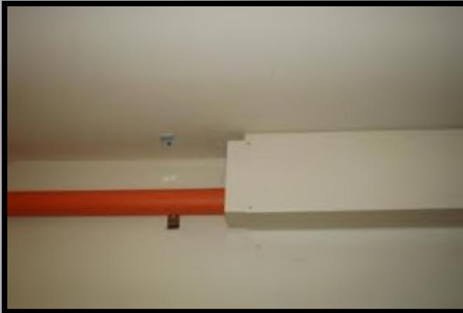
6. SLIDE ADJACENT SECTION OF MATERIAL OVER COUPLING
