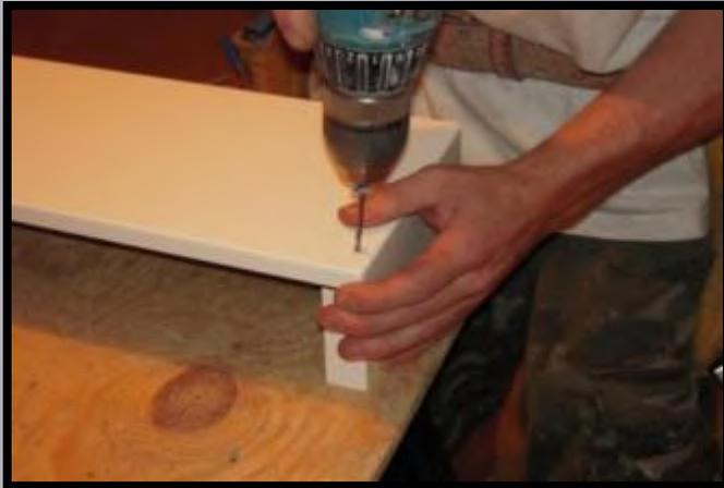
2. AFTER A FLUSH ALIGNMENT, RIVET END CAP INTO PLACE
