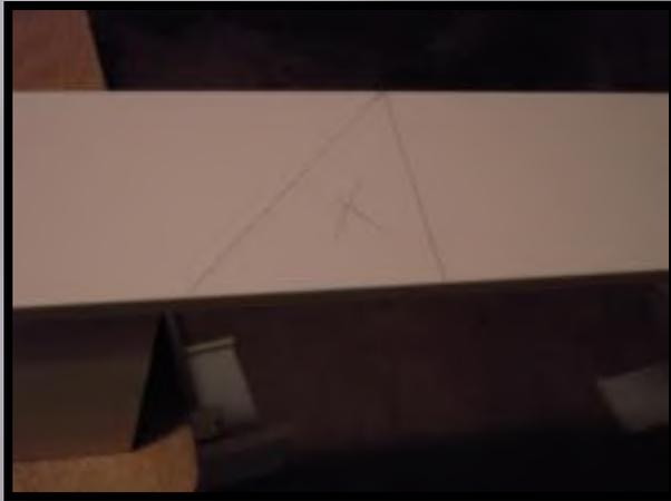
2. NOTCH A "V" INTO THE EDGE OF YOUR PIPE ENCLOSURE
